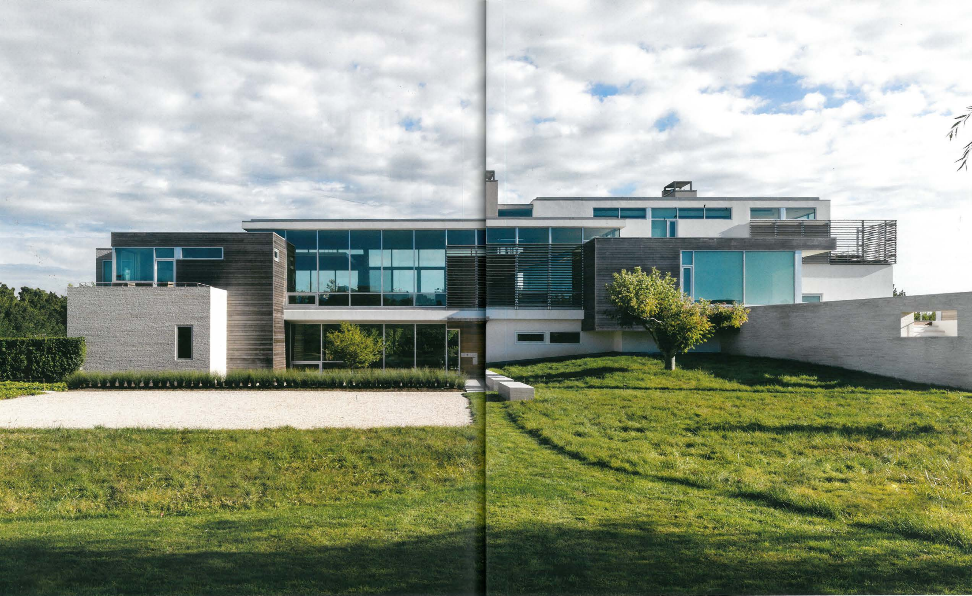
THE FRONT VIEW OF THE 10,000-SQUARE-FOOT HOUSE IS A CAREFULLY LAYERED COMPOSITION OF OPEN AND CLOSED VOLUMES RISING FROM THE EARTH TOWARD THE SKY. SOLID HORIZONTAL STONE ELEMENTS AT EITHER END ANCHOR IT TO THE GROUND, WHILE STUCCO, CEDAR, AND GLASS FORMS RISE IN EVER LIGHTER COMPOSITIONS TO THE TRANSPARENT BRIDGE THAT COMPRISES THE MAIN LIVING SPACES.
